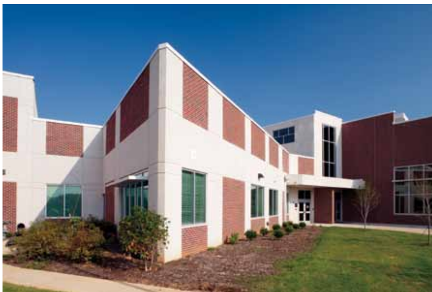
The classroom design was modified from a straight wall to a sawtooth design that ensured that each room featured fenestration that opened to the southwest or southeast.
