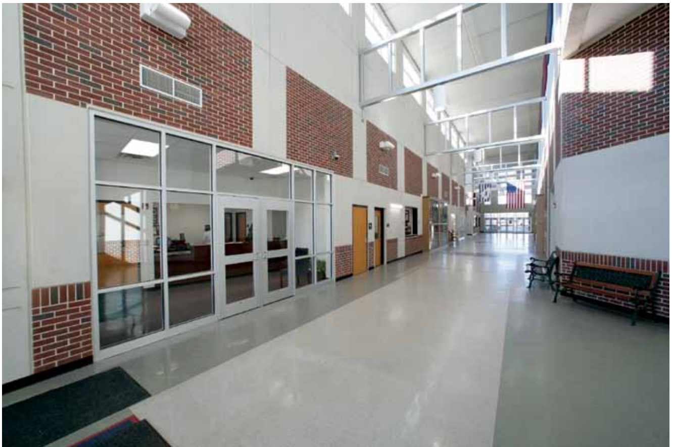
Thin brick embedded into the architectural panels used both for interior and exterior facings replicated the color and texture of those used on the original high school.
