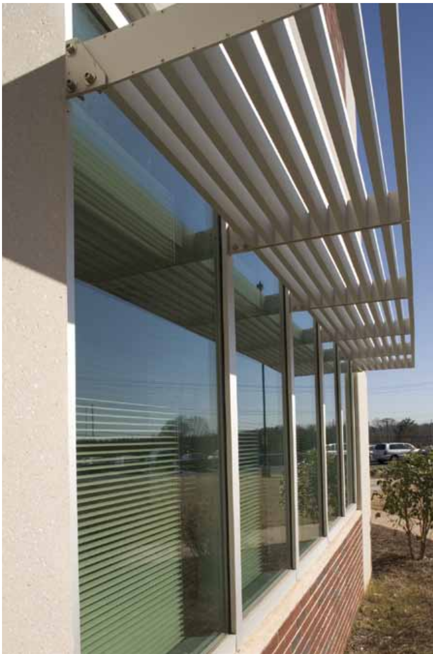
Solar shields above windows help control daylight to ensure rooms stay bright but don't become too sunny or hot.
